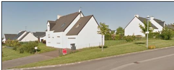
Habitat individuel – Ossé Source : Google Street View
